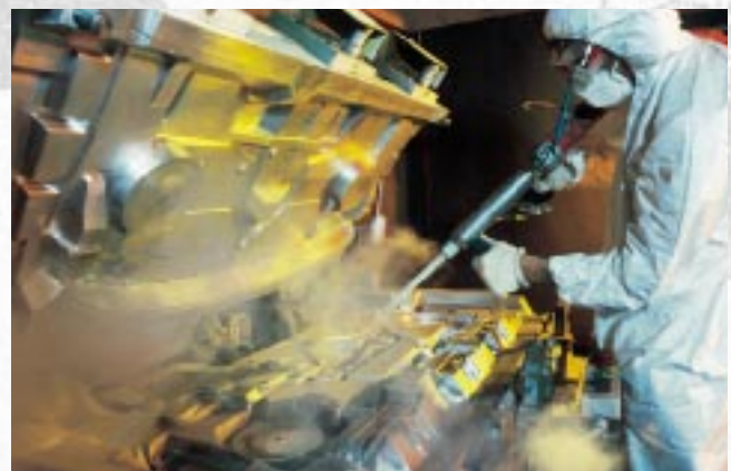
Surface cleaning with the mobile dry-ice blasting system CryoMax®. Linde's effective and environment-friendly alternative to conventional cleaning processes.
